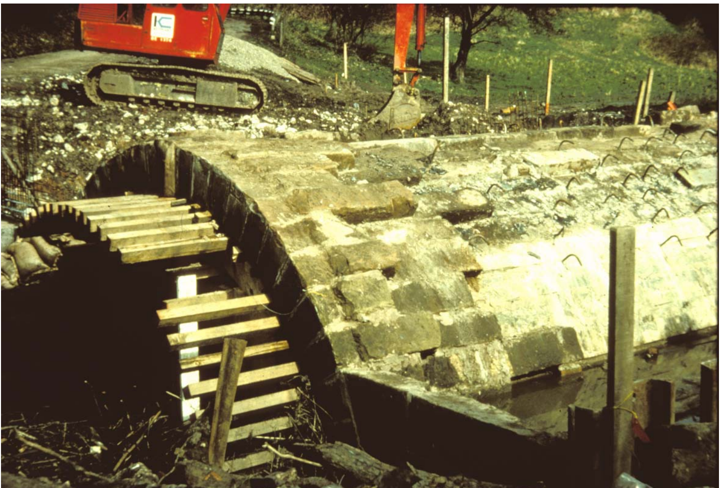
Rebuilding the old bridge to allow passing traffic- 1978
