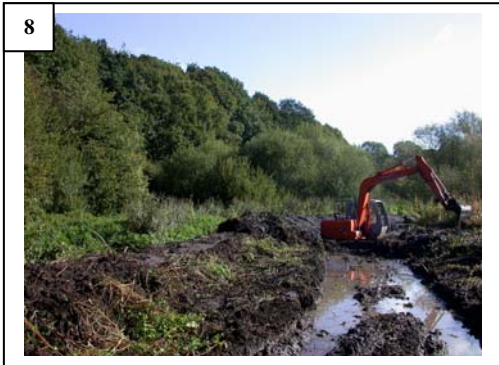
Making the bund to pond the flood water
