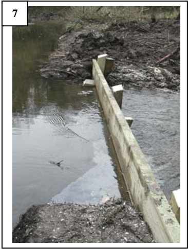
Small weir construction where the ditch join the river
