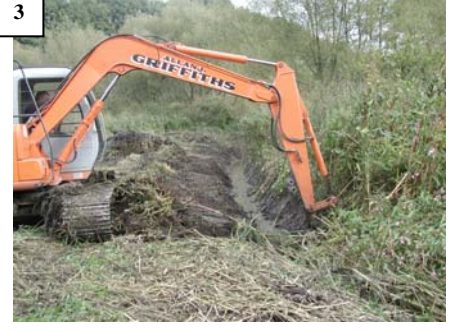
The old ditch being dug out and broadened for 'lagoons'
