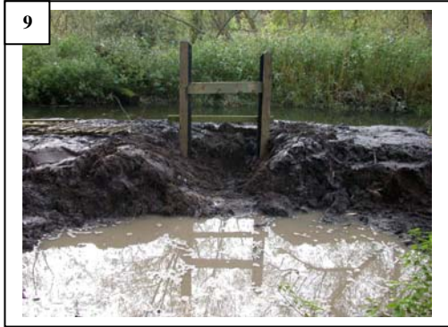
Building of a sluice gate in place of the small weir
