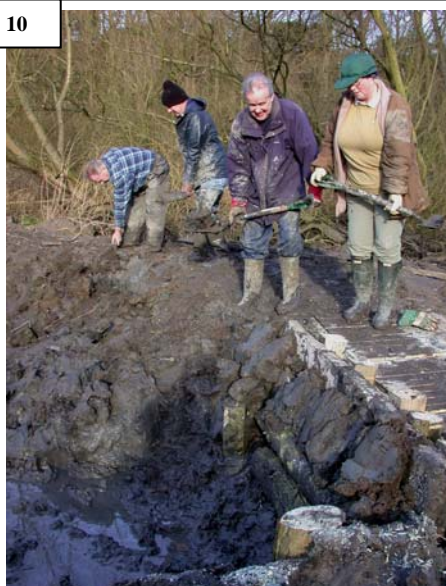
Weir constructed downstream to stop water escaping from Babbs Meadow
